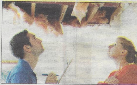
Asbestos falling from the ceiling could be a reason to sue.
